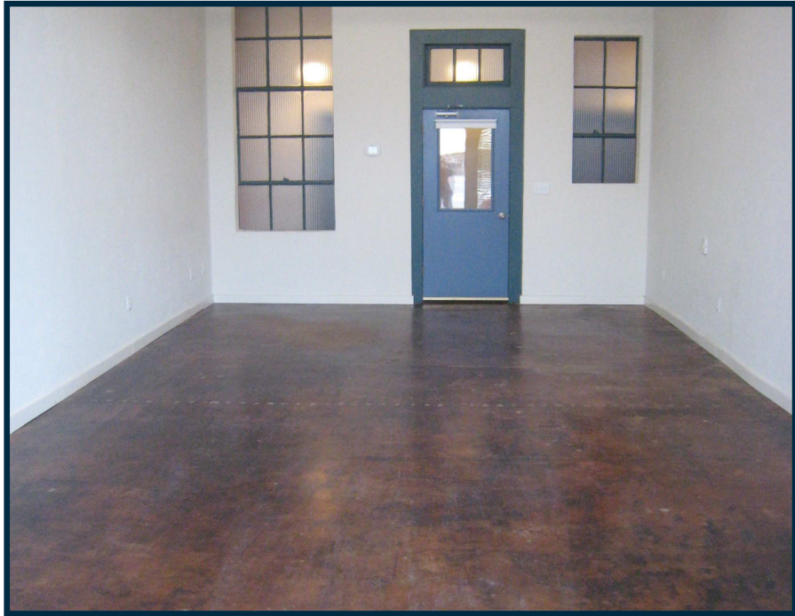
Original Interior View
